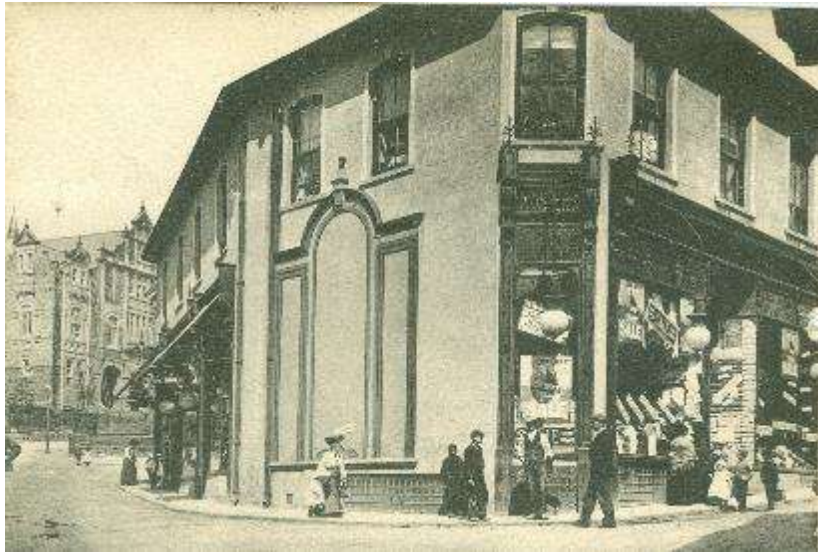
Left: the rebuilt Blaenavon Co-operative Stores, Blaenavon (c.1902).
