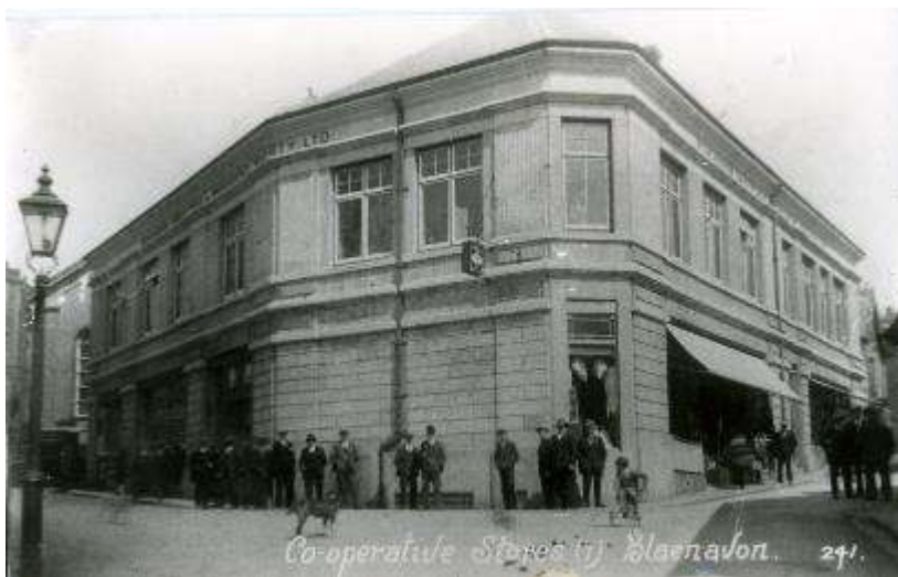
Left: the fire of 1918 necessitated another rebuild. The new stores were opened in 1928.
