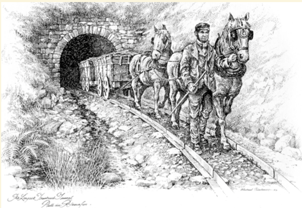
One of the entrances to Pwll Du Tunnel. At 2 kilometers (1.2 miles) in length this was the longest tunnel on any horse-drawn tramroad in Britain. Illustration by Michael Blackmore.
