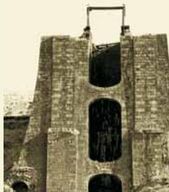
Wales, and remains of the iron hoist survive. The water balance was used to lift iron and raw materials in trams between the furnace tops and the yard area below. It was built in 1839 as part of a modernisation programme by James Ashwell, managing director of the Blaenavon Iron & Coal Company. The Ironworks site is open to the public from April to October. Telephone (01495) 792615 for further details.
