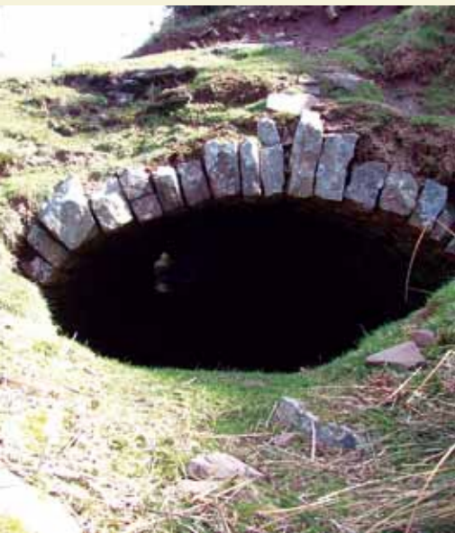
'Cut & shut' tunnel entrance
