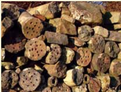
Wall built with Bessemer ‘Tuyeres’ at Bunkers Hill
