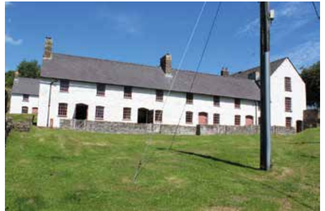
STACK SQUARE, BLAENAVON IRONWORKS
