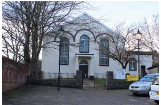
BETHLEHEM CONGREGATIONAL CHURCH (ALSO KNOWN AS BETHLEHEM INDEPENDENT CHAPEL), BROAD STREET (W SIDE)
