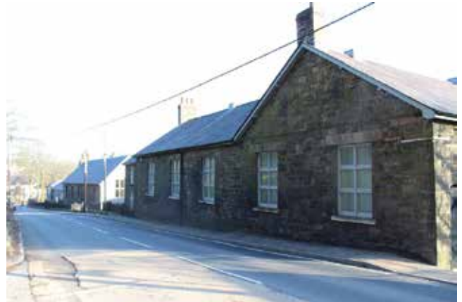
FORMER ST PETER'S BOYS' SCHOOL (NOW RAMFIELD STUDY CENTRE), CHURCH ROAD (SW SIDE)
