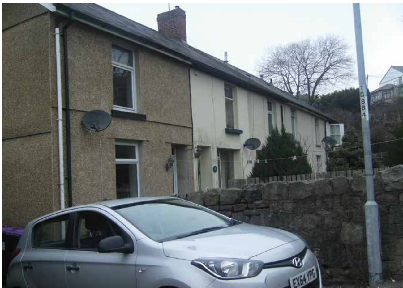
Loss of chimney stacks and pots, windows and doors with inappropriate wall finishes change the character and design of this traditional terrace.
