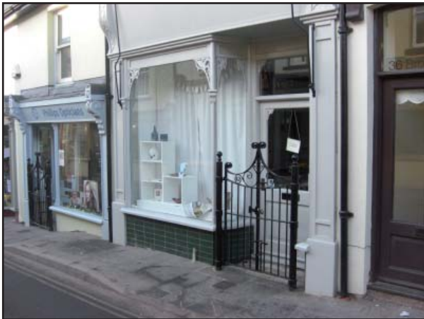
Recessed doorways can be secured with wrought iron or steel gates.
