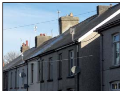
Where chimney pots have been removed the roof profile loses an important part of its consistency and regularity of rhythm.
