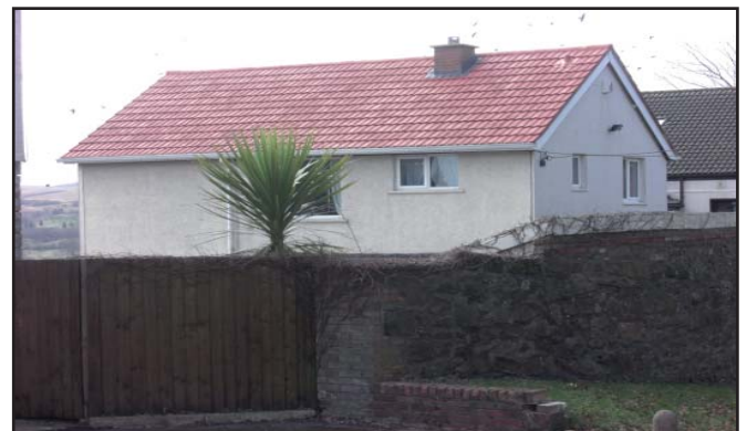
Brightly coloured tiles are particularly alien to the palette of materials and natural tones of the landscape and traditional buildings in the WHS, are unacceptable and should be avoided.
