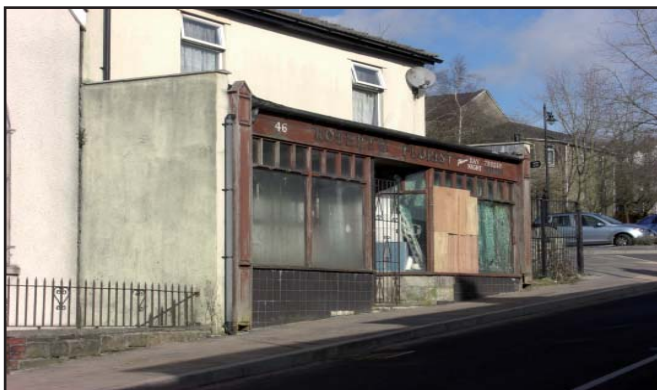
Buildings in a poor state of repair have a detrimental impact on the wider area.
