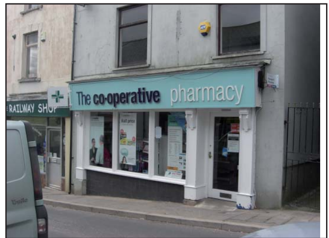
The fascia should not be too large, as in this example in Broad Street, to avoid an imbalance of proportions and over-dominance of the elevation as a whole.
