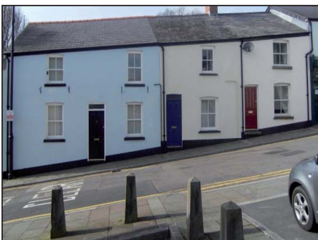
In some parts of the WHS, the roofs of the terraces are sloped rather than stepped. The double fronted dwelling on the left illustrates the way that larger properties could be integrated within the terrace whilst still maintaining the overall rhythm and character of the streetscape.
