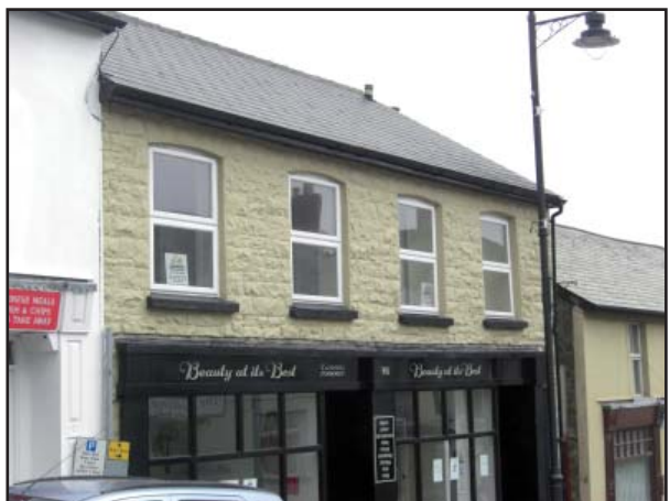
Natural stone should not be painted under any circumstances. It can lead to the disintegration of the stone and is likely to cause greater problems and costs in the long term.
