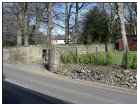
Stone boundary walls form an important component in the streetscape of the area and should always be retained. Hedges and timber fences do not provide the same character and qualities, particular to the WHS area.
