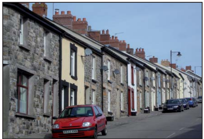
Many of the terraces are built directly on the back edge of the pavement, providing a strong and robust edge to the streetscape.
