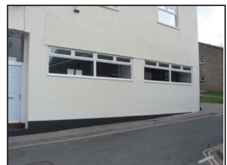
The vertical emphasis of the windows openings is an important part of the character of the area. Horizontal designs look completely out of place and should be avoided.
