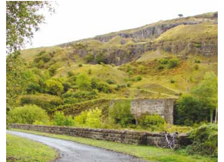
Clydach South Station
