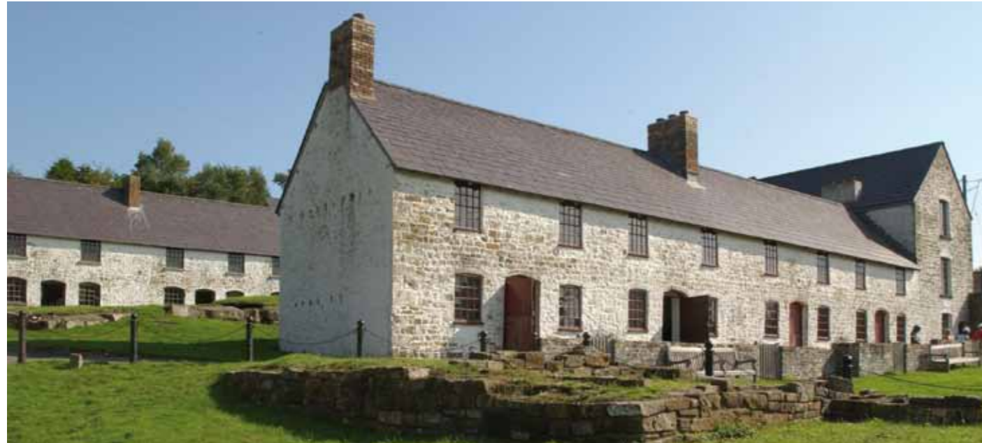
Stack Square, Blaenavon Ironworks, where the families will live
