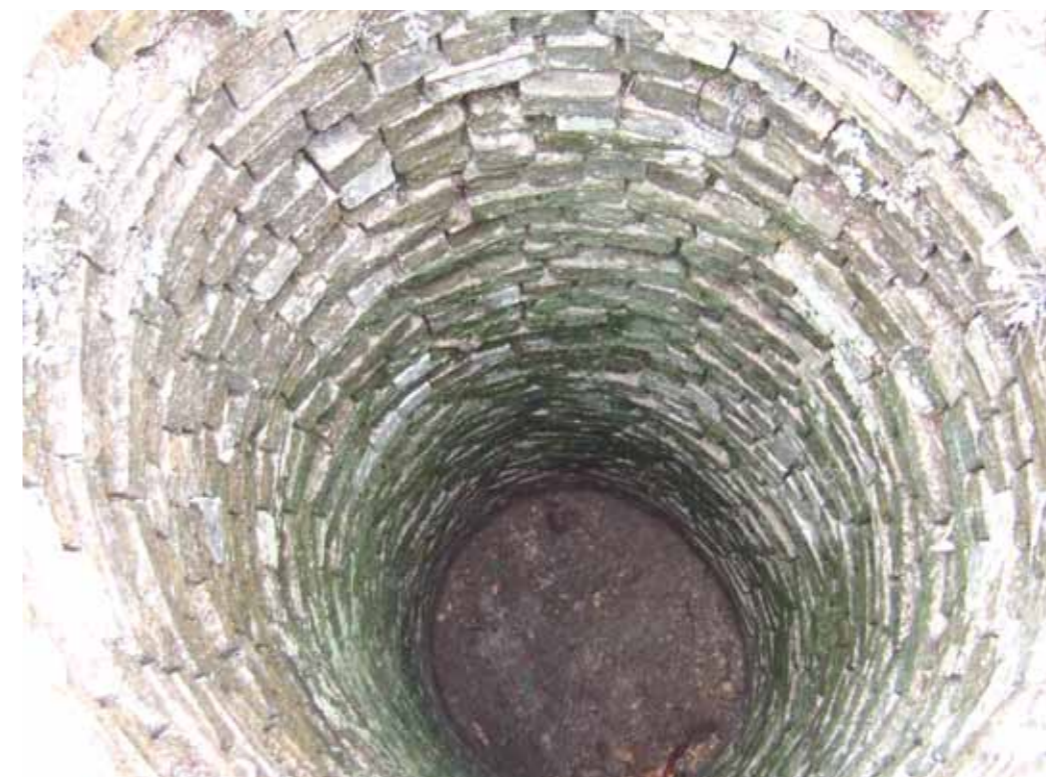
The chimney interior following restoration © TCBC
