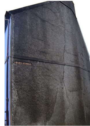
Above, left: Cracks in cement render
