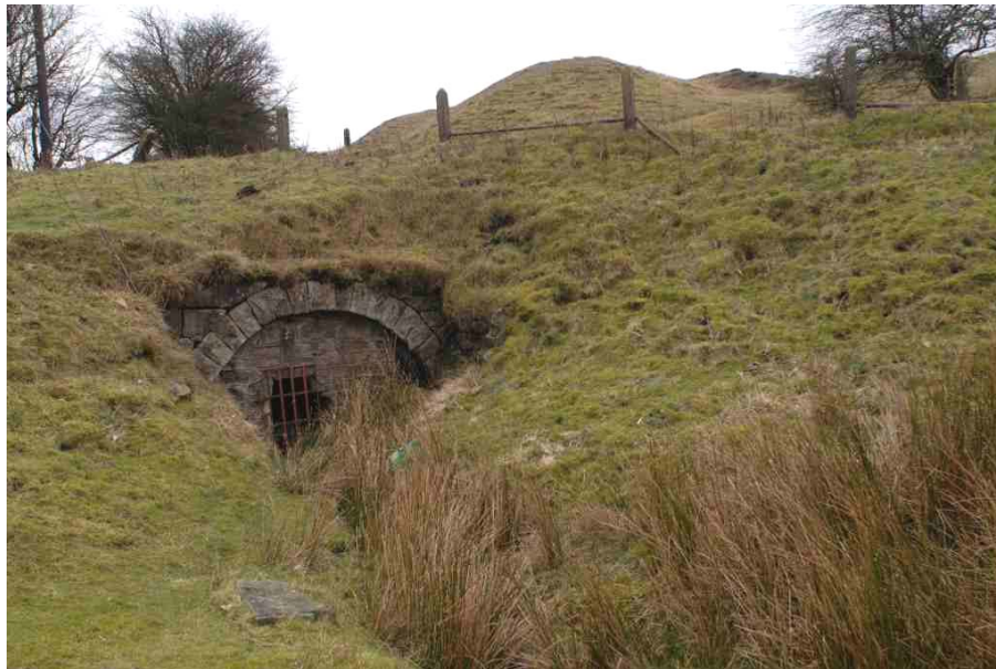
Entrance to Pwll Du tunnel RKE
