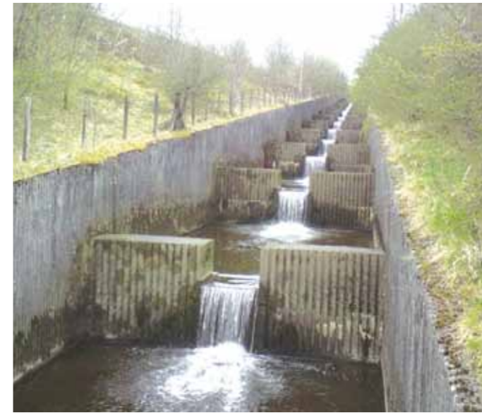
Micro hydro scheme will be installed at the Dragon's Teeth on the Afon Lwyd
