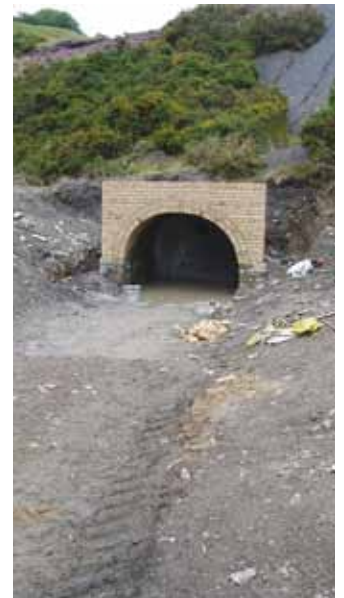
Restoration to the southern portal of the Pwll Du Tunnel
